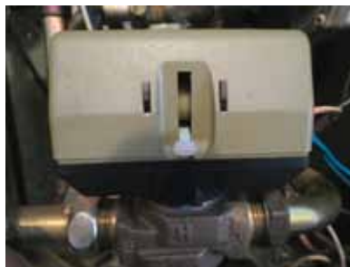
Driewegklepcartridge in cv-stand
