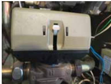
Driewegklepcartridge in ww-stand
